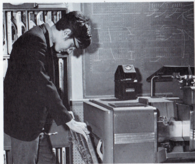
Anxious to see the results of his wiring, Gerard Joria inserts the control panel in the 402 accounting machine.
